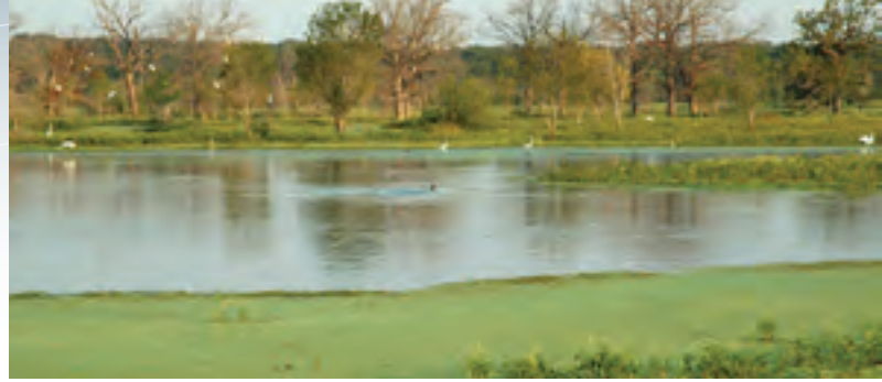
TRWD wetlands water reuse project Photo courtesy of Tarrant Regional Water District
