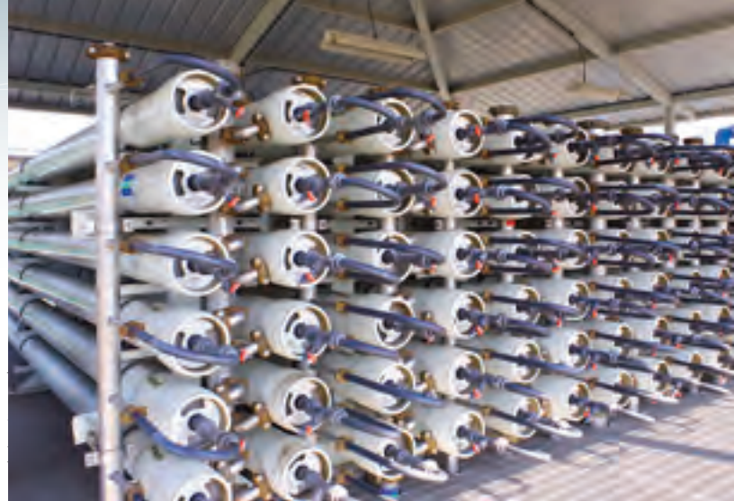
Reverse osmosis membranes used to help stop seawater intrusion and replenish local groundwater basins Photo courtesy of the Water Replenishment District of Southern California
