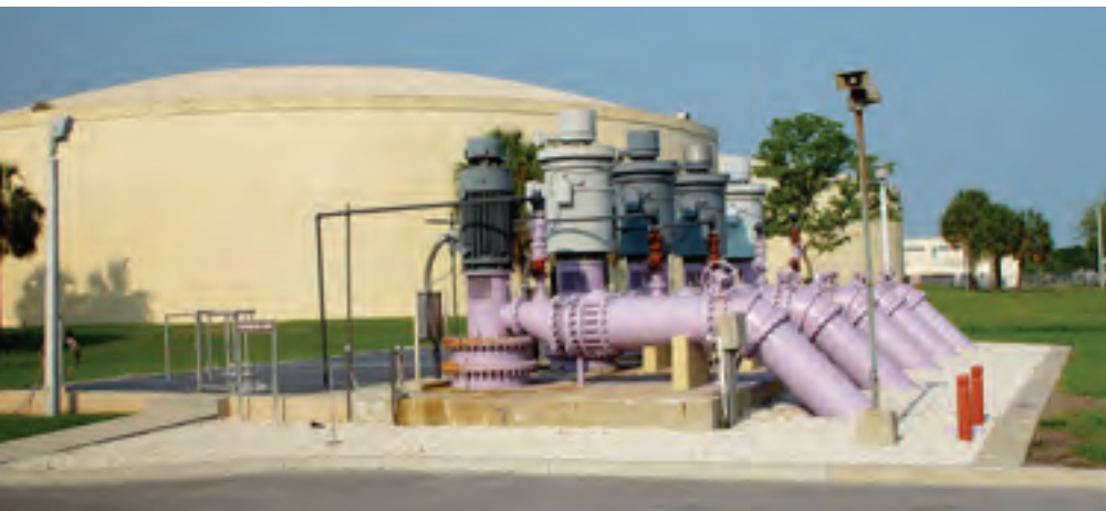
Northwest Water Reclamation Facility
